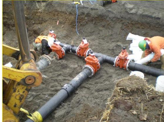
New HDPE pipe was attached to the back of the expander head, replacing the line.
